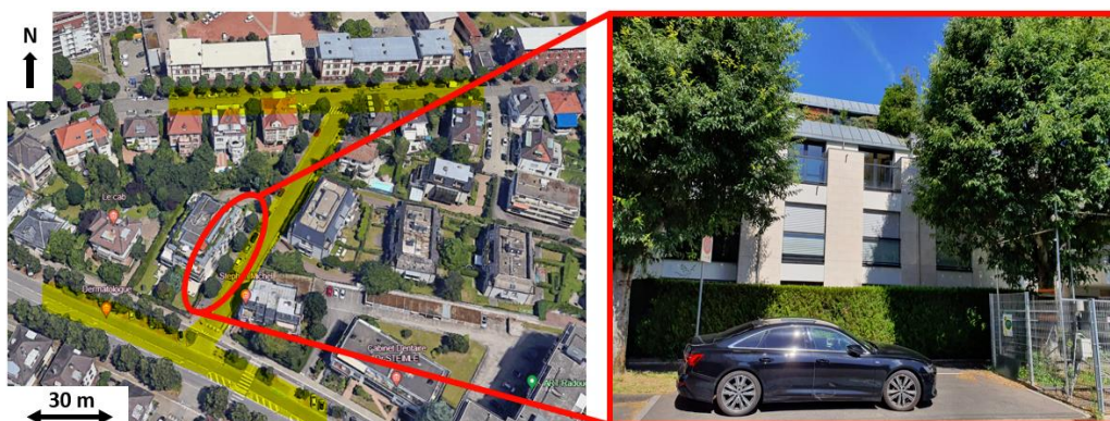
Figure 1: Study area in Strasbourg (left) and the main facade under study (right). The three streets are highlighted in yellow (Source: Google Earth)
